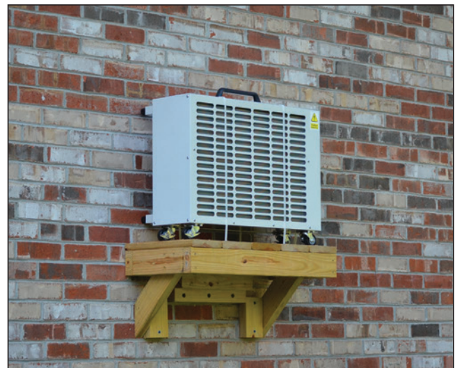
Outdoor Heat Exchanger* *does not need to be mounted off the ground
